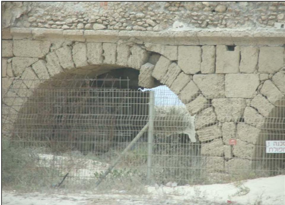
**Figure 8: Closeup of structure of reconstructed ancient aqueduct nearby GPR Survey area, and potentially fitting the characteristics of the anomalies found in Grid 1 and Grid 3.**
