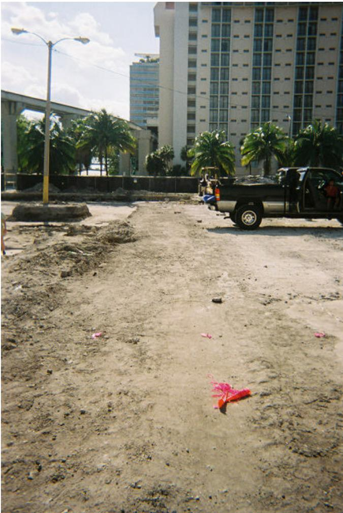
Within the grid, which was marked out in the dimensions of 21 meters (East-West) by 4 meters (North-South), GPR signal data was acquired in a tight set of 21 overlapping parallel lines taken first East to West, and then transected by 20 lines in a perpendicular direction North to South subset grid (Dataset 2). Dataset 2 was located from 3.5 – 7.5 meters along Dataset 1.
